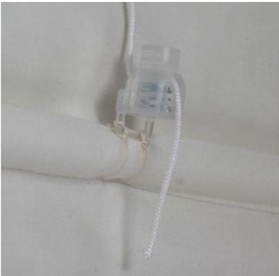
The rear cords or tape on the blind should be connected to the blind using a safety breakaway system.
